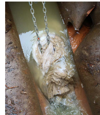
Our domestic misuse 'hedgehog' devices will help to tackle blockages by capturing and removing unflushables, evidencing the scale of the problem.
