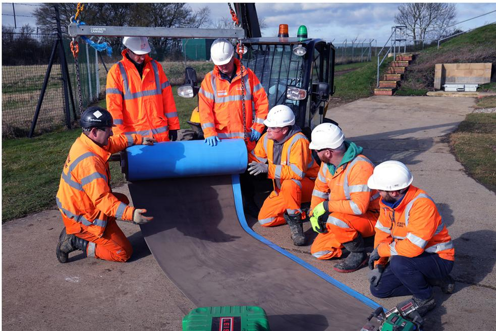
Trialling concrete canvas at our Gazeley Water Treatment Works in Suffolk: this is a much quicker and significantly more carbon-efficient method of laying concrete.
